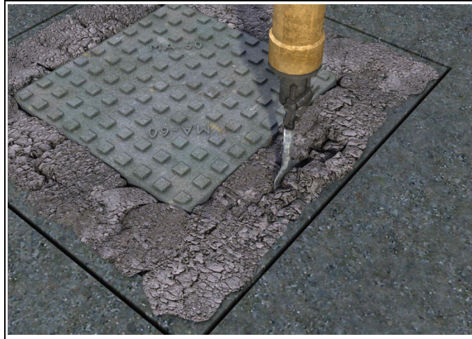
Figure 2 Excavating failed ironwork
