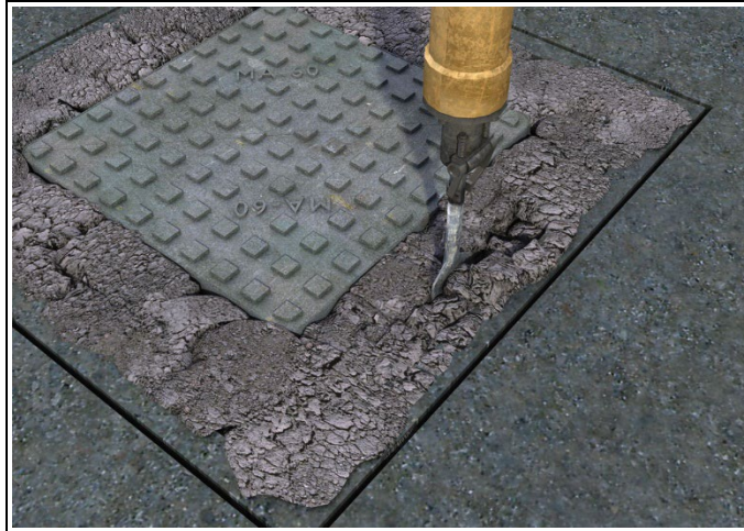
Figure 2 Excavating failed ironwork
