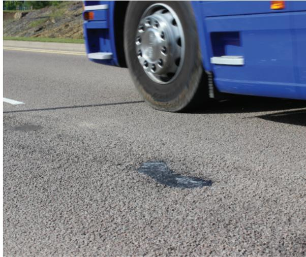
A surface defect repair system developed to address specific areas of preventative maintenance.
