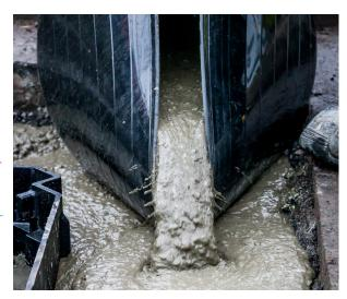
A fibre modified concrete for backfilling around manhole frames and gullies and can also be used for surface repairs.
