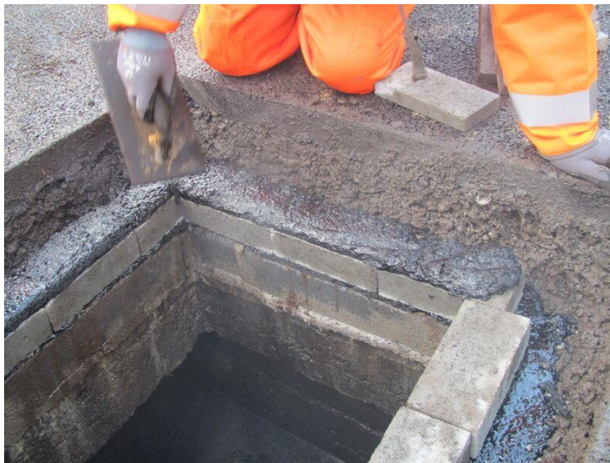
Installing second layer of polymer modified mastic asphalt as bedding
