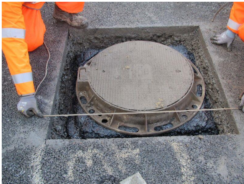
Placing frame and cover
