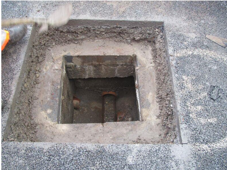
Manhole chamber top exposed
