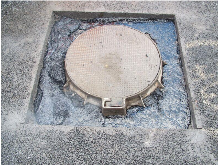
Polymer modified mastic asphalt placed as binder course
