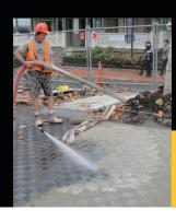
Instarmac's New Zealand partner, Horizon International Paving, have supplied UltraScape Pro-Bed HS and Flowpoint to install and grout granite setts on a busy bus lane in Auckland.
