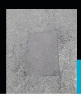
Highway, engineering and construction specialists, Cormac Solutions Ltd., have used UltraCrete Tough Patch Rapid® to repair a number of potholes throughout Cornwall.
