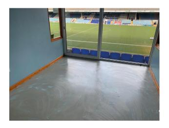
Developed for the renovation of existing floors, Level IT Renovate is fibre reinforced for added strength and to minimise the risk of hairline cracks – reducing a common cause of failure.
