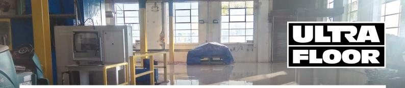
To complete the installation, the cured floor was then prepared by industrial grinding before the application of two coats of a solvent free epoxy coating – resulting in a flat, hard-wearing, safe and fit for purpose floor.
