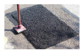
Tough Patch® is a PTS PAS approved, cold lay surface material for road repairs, which utilises a reactive binder that rapidly cures to create a first time, permanent repair that will accept traffic immediately after installation. By ultilising Tough Patch®, the amount of time needed for closures on a highway can be reduced, resulting in a significantly safer working environment for the Keir operatives carrying out the work.
