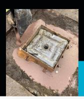
Leading UK utility contractor, Telent, have used UltraCrete's superb ironwork installation materials to repair and install a CW1 access cover in Sutton Coldfield.
