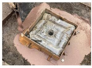
Flowable high performance bedding mortar is BT LN550 and LN320 compliant and offers superior compressive, tensile and flexural strengths in just 3 hours.
