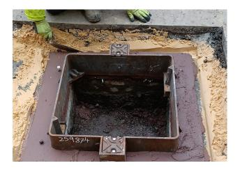
Once in position, Envirobed® CD534 Red high performance bedding mortar was applied to the inner face and chamber top and the timber shuttering was then placed 50mm beyond the flange.
