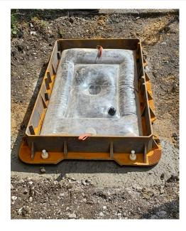
HT Installations Limited utilised UltraCrete QC10 F flowable fibre modified concrete to repair the brickwork chamber and their Envirobed® Flowable Installation System to install the replacement CW2 frame and cover – a process used by Openreach for all their carriageway repairs.
