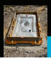
UltraCrete's market-leading Flowable Installation System has been used to repair a faulty carriageway frame and cover on the B4299 in Carmarthen.
