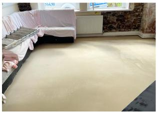
system for use as a surface damp proof membrane. Designed to provide protection against subfloor moisture, DPM IT has a pot life of 45-75 minutes, a cure time of 5 hours and boasts a 98% RH floor moisture tolerance.
