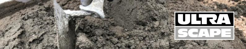
To complete the installation, flowpoint rapid set flowable grout was used to joint the selected pavers. UltraScape flowpoint is a flowable grout which allows for large areas of paving to be grouted quickly. Suitable for joints from 3mm to 50mm and as deep as 200mm, flowpoint has been developed over a number of years to provide a durable finish which will not crack or stain - even in the extremely hot and cold temperatures.
