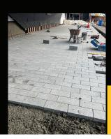
UltraScape's BS 7533 Mortar Paving System has been used to install 780sqm of paving and 200lm of kerbs at Tākina Wellington Convention and Exhibition Centre.
