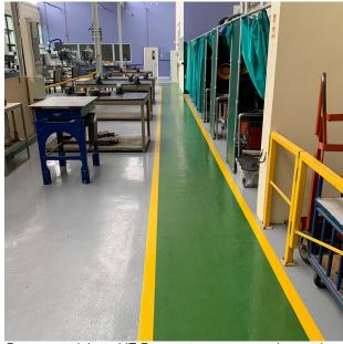
Once cured, Level IT Renovate was poured over the concrete substrate at a depth of 40mm.
