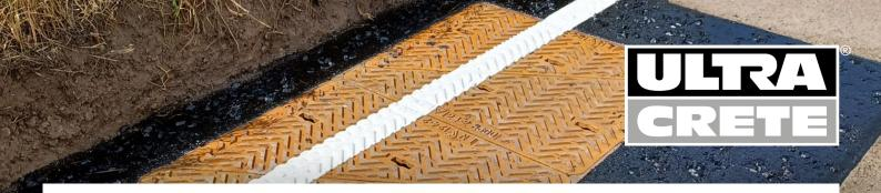
UltraCrete Enviro Mastic® was applied by the contractors in standard layers and stone chippings added to the final wearing course. To complete the project, the reinstatement was overbanded to seal the old and new surfaces and road markings replaced using Instaline in white.
