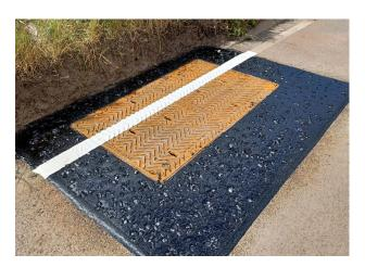
was levelled with the existing road surface using a string line and Install Plus levelling feet with external shuttering placed to retain the flowable mortar 50mm beyond the flange edge. To further reinforce the shuttering and prevent any seepage, a sand bund was applied behind the shuttering. Once in place, a carriageway 2 Mortar Buoy® was inflated to seal the chamber top and frame ahead of the mortar pour.
