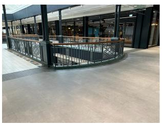
To begin, Specialist Flooring Group's screeding team installed UltraFloor Screed IT UltraCem fibre modified cement binder across the 1800sqm area, before handing over to their flooring division to carry out the remainder of the subfloor preparation, by trowel applying UltraFloor Level IT Hydra Bond up to 5mm.
