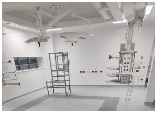
the application of Marmolium and sheet vinyl floorcoverings, the Puma Flooring team utilised UltraFloor's DPM IT damp proof membrane, Prime IT Multi-surface Primer and Level IT Two multi-purpose floor leveller.
