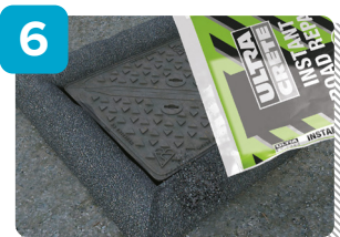
Surface finish with UltraCrete Instant Road Repair or Tough Patch cold lay asphalt concrete if located on a footpath, or category 3 & 4 road.
