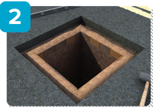
Old bedding mortar, loose bricks and debris are removed.
