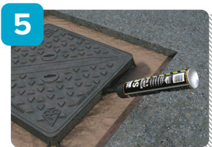
UltraCrete SCJ edge sealant and bitumen tack coat should be applied to all edges of the trim back and new frame.
