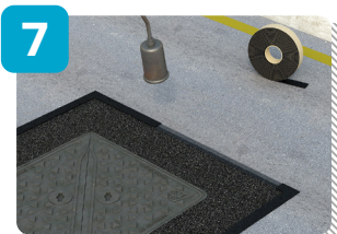
Once the surface course is compacted, apply UltraCrete Instaband ECO® thermoplastic overbanding to the edges of the reinstatement.
