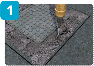
A picture frame is saw cut and excavated and the existing cover and frame removed.
